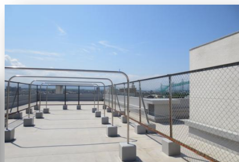
↑Roof (for laundry)
